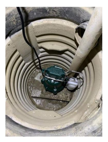
• Sump Pump Cleaning and Inspection: Our experts will clean out your sump pump pit, check for debris, and inspect key components like the check valve and backup battery to ensure everything is in working order.
