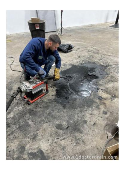
6. Floor Drains Backing Up: If you're noticing your floor drain is backing up, it's likely due to a blockage or a damaged pipe. Floor drains are essential for draining water away in basements, laundry rooms, and other low-lying areas, but they can easily become clogged with debris or even suffer from issues within the main sewer line. Doctor Drain's technicians can diagnose the cause of your backup and implement the right repair solution to restore drainage.
