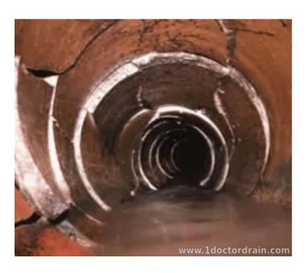
3. Broken or Shifted Pipes: Pipe shifting often occurs due to ground movement, settling soil, or heavy traffic above the ground, like cars or construction equipment. This can cause joints to disconnect or pipes to crack. Broken or shifted pipes need careful repair to prevent leaks and ensure proper drainage. At Doctor Drain, we assess the damage and perform the necessary repairs, using techniques that can minimize the impact on your property.
